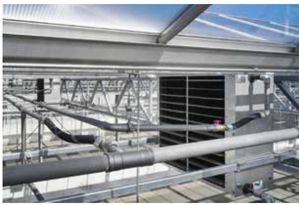
The incredible strength of the steel pipes and the Megapress connection pieces means piping can be installed below the hall ceilings with a minimal number of fixed points.
