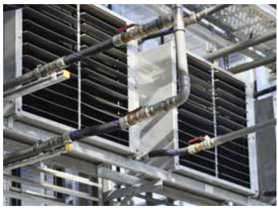
Flexible, to compensate for movements caused by thermal and mechanical influences: The connections to the heating coils and to the main distribution system.
