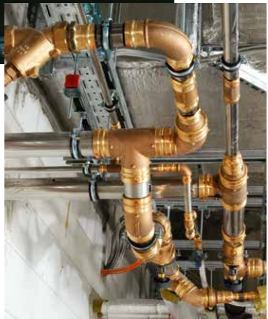
A total of 8 kilometres of Sanpress stainless steel piping was installed for the main drinking water distribution system.
