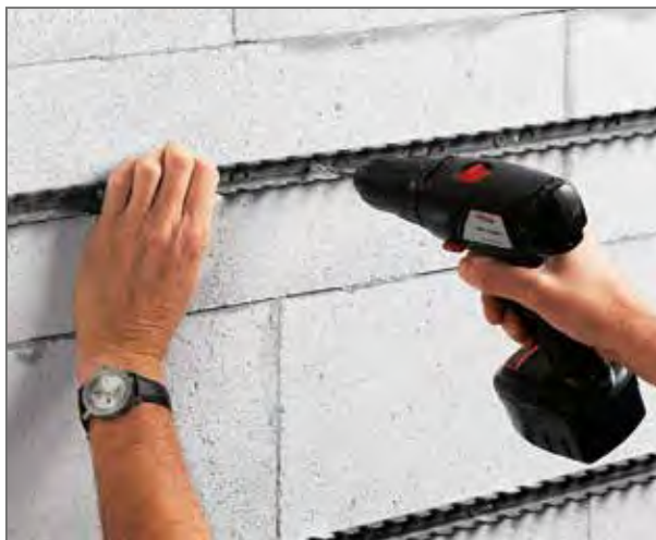
Fig. 186: Fastening the clamping rails
