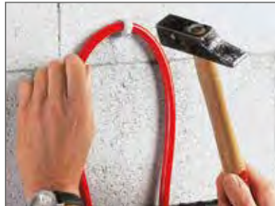
Fig. 188: Fastening in curved sections
