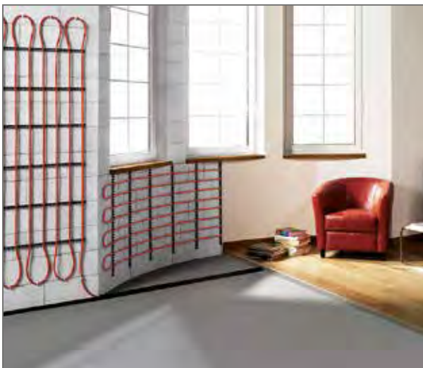
Fig. 178: Installation situation Fonterra Side 12 Clip
