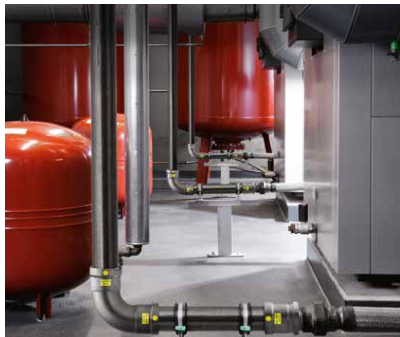
Safe transport for inflammable media – metal Viega press connectors make it possible.
