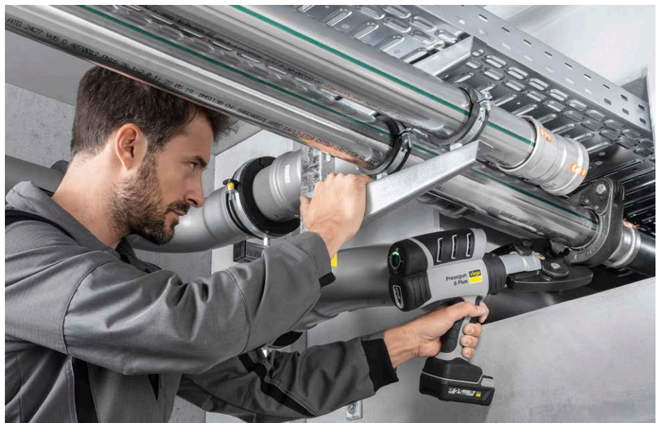
Even hard-to-reach connections can be easily pressed with the Viega press rings and hinged press jaws.
