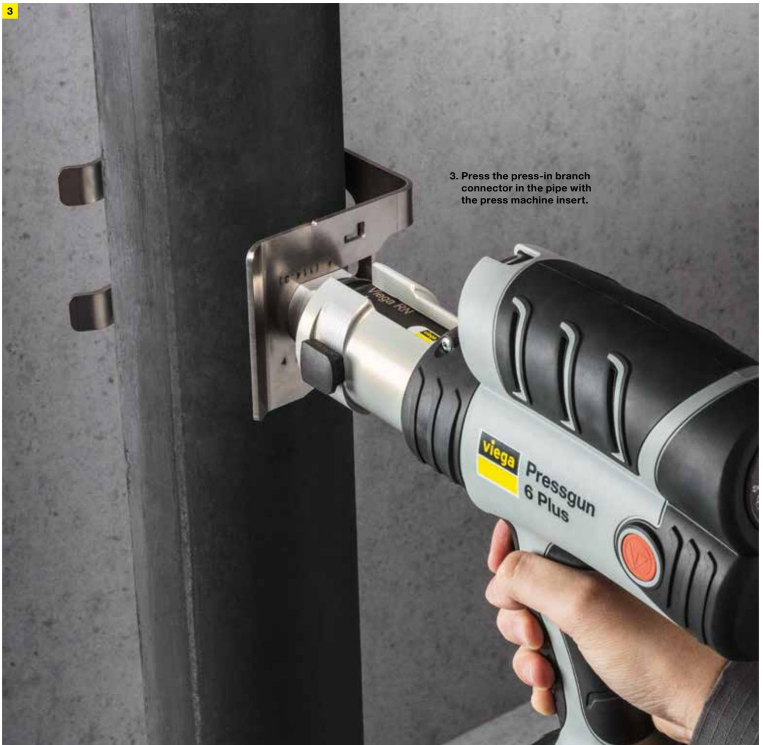
3. Press the press-in branch connector in the pipe with the press machine insert.
