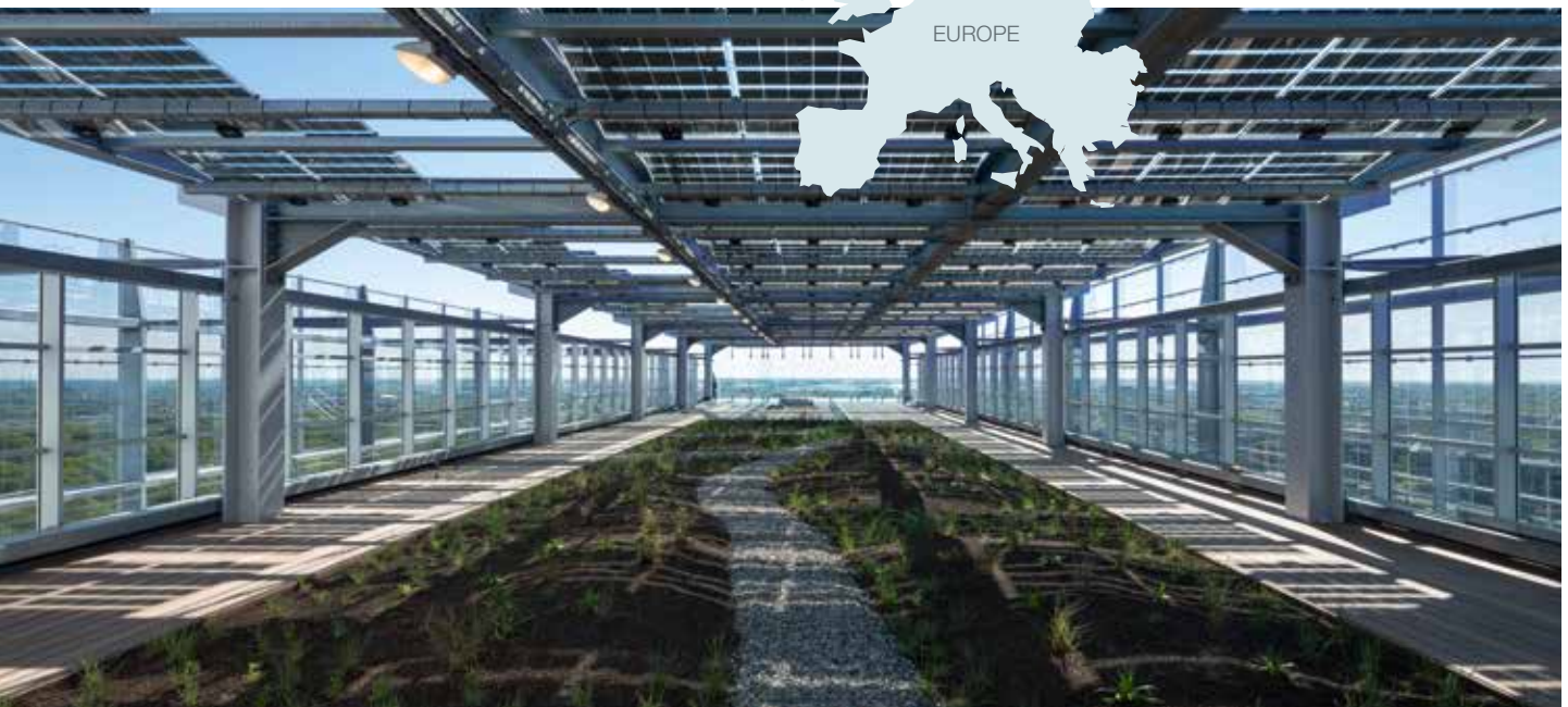
© Photo: Ossip van Duivenbode. Commissioned by European Patent Office
