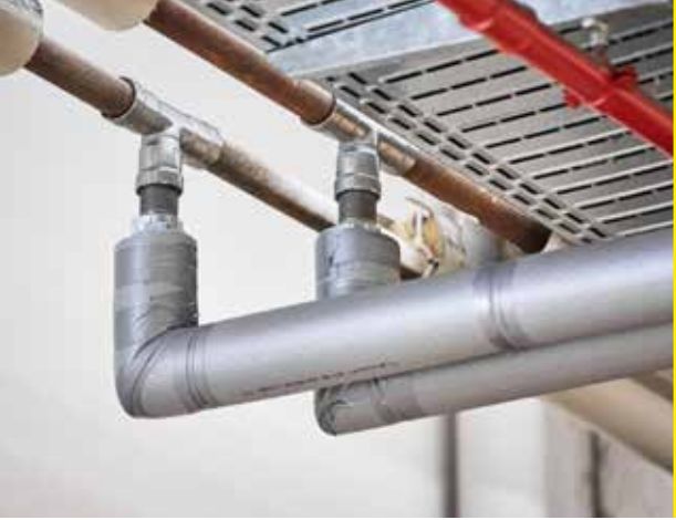
Pressed in seconds rather than laboriously welded: Megapress outlets in the production hall.
