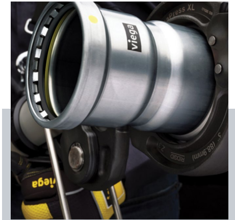
Press Connection (Viega Megapress)
