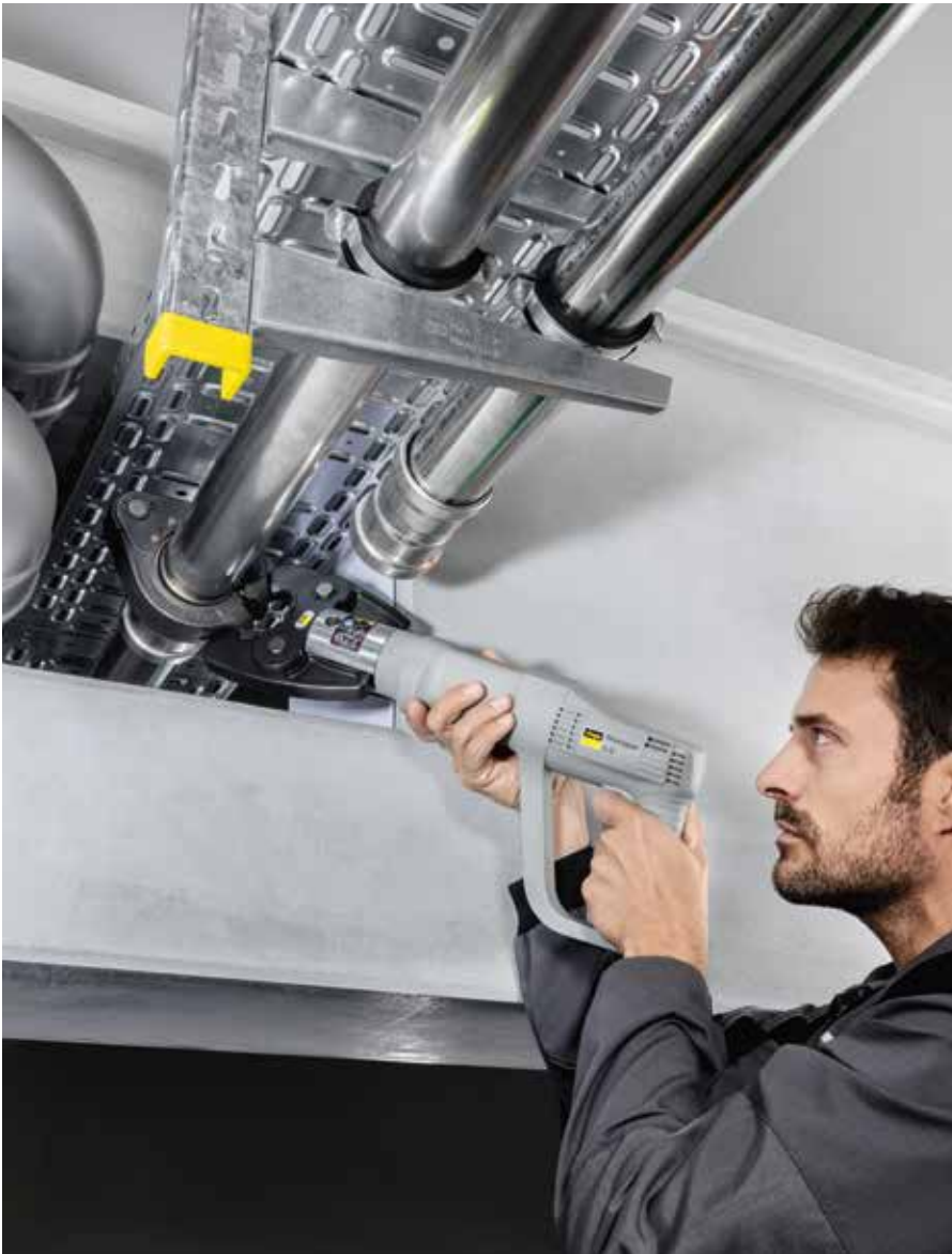
Compact, light and high-performing: the Viega Pressgun 6 B offers exceptional handling.
