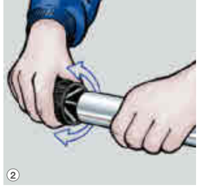
② De-burr pipe internally and externally.
