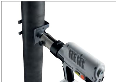
Fig. 147: Press the press-in branch connector to the steel pipe. The pipe outlet has been created.
