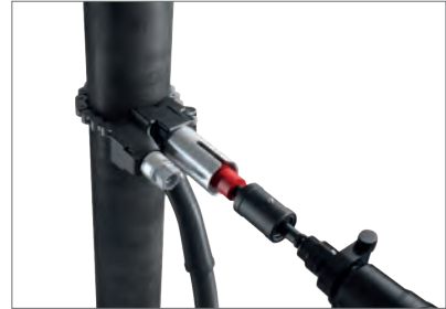
Fig. 146: – Drill into the steel pipe (Fig: Steel chips are suctioned away) – Disassemble the holding device
